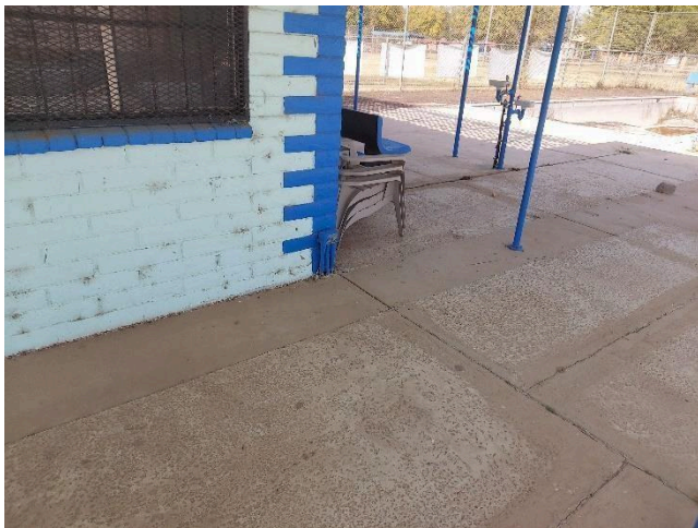
Electrical junction box – not elevated above pool water surface to comply with NEC.
