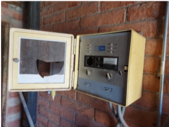
Storage room – debris and trash restricting access, inoperative equipment, electrical equipment does not have sufficient clearance to comply with NEC.
