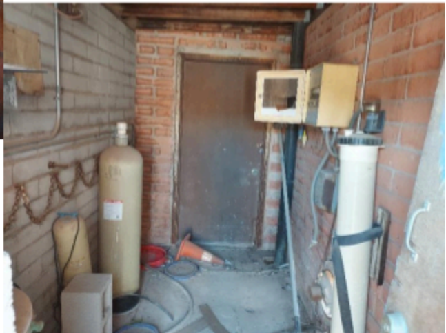
Storage room – debris and trash restricting access, inoperative equipment, electrical equipment does not have sufficient clearance to comply with NEC.
