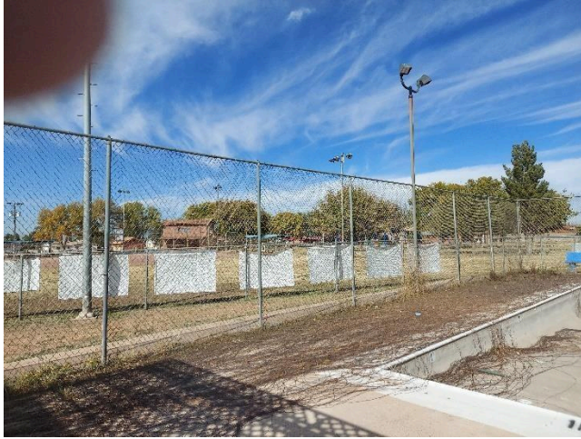
Chain link perimeter fence and exterior pole lighting.
